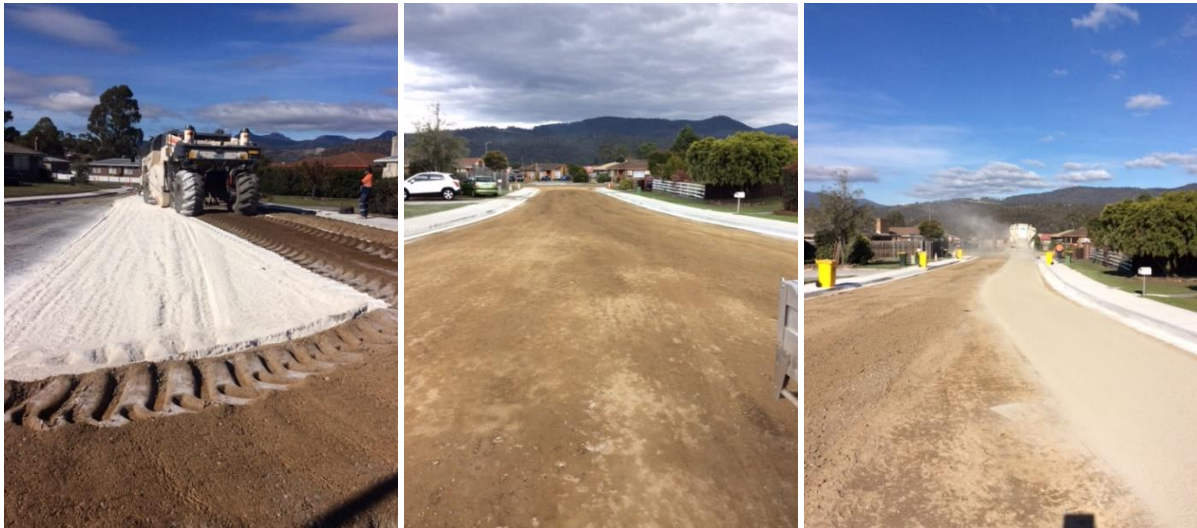
Figure 30. Basegrade Stabilisation, Schoobridge Place, New Norfolk, TAS (Goodsell, 2020) 3% Lime Treatment (L); 24 Hour Curing Period (Middle); 3% Cement Treatment (R)
